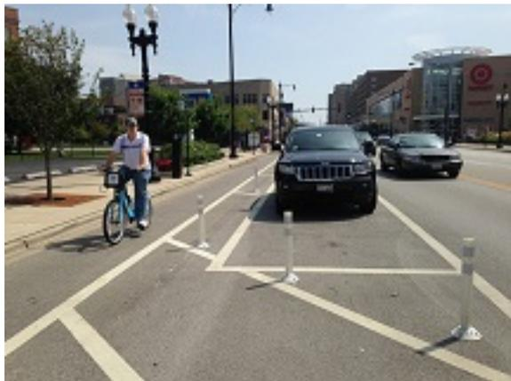
**Buffered bike lanes:** Are designated by a white stripe, a bicycle symbol, and signage that alerts all road users that a portion of the roadway is for exclusive use by bicyclists. The presence of a striped, horizontal buffer (greater than or equal to 18 inches) provides additional operating space and lateral separation from moving and parked vehicles.
